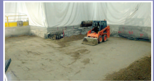
Filling of excavation
