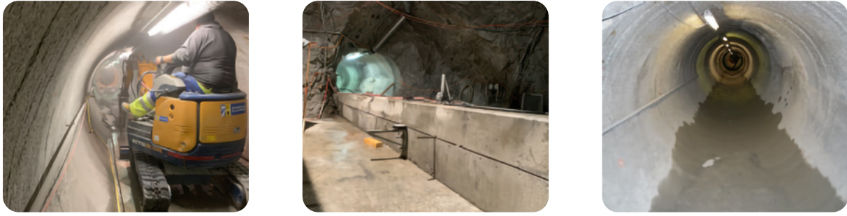
Figure 5-28: Gallery of the Grimsel underground laboratory (Nagra)
