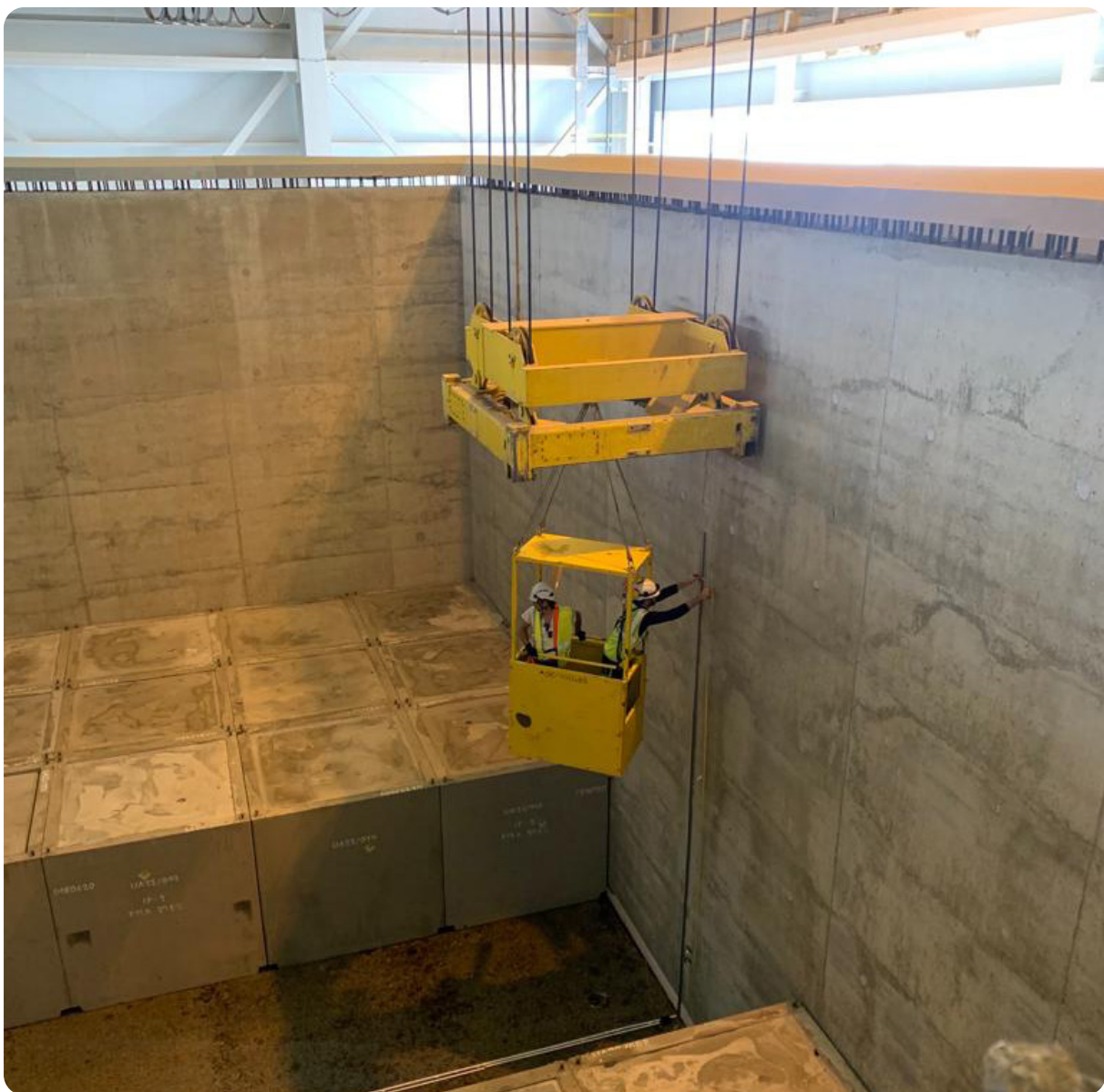
Figure 4-1: Installation of sensors in Vault 21 at El Cabril Disposal Centre
