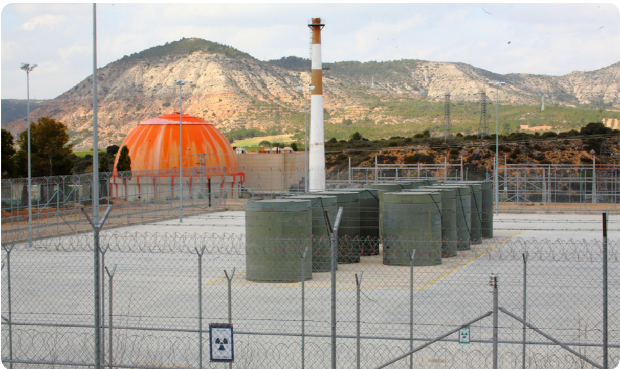
Figure 4-5: General view of the ITS at José Cabrera NPP
