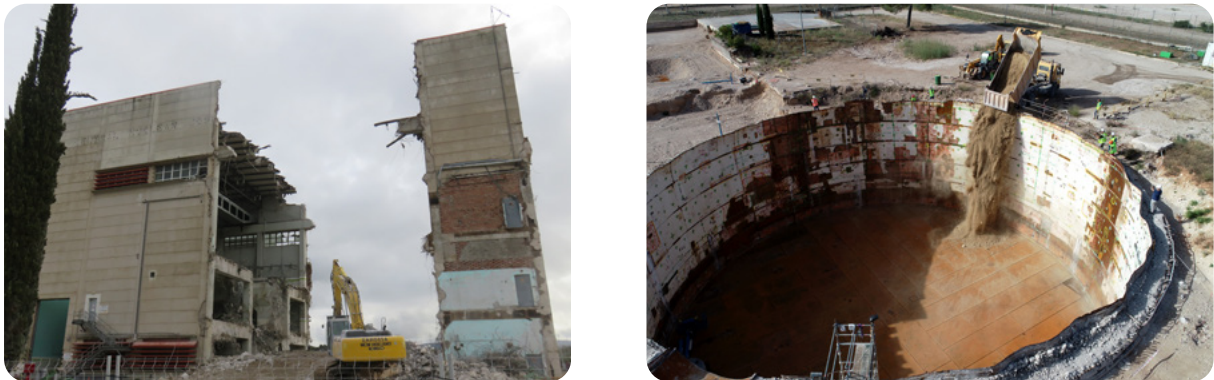
Figure 3-15: Different phases in the decommissioning of José Cabrera NPP
