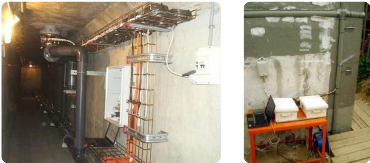
Figure 5-31: Data acquisition system in the infiltration control network gallery of Vault 1; data acquisition system of Vault 16 during the assembly phase
